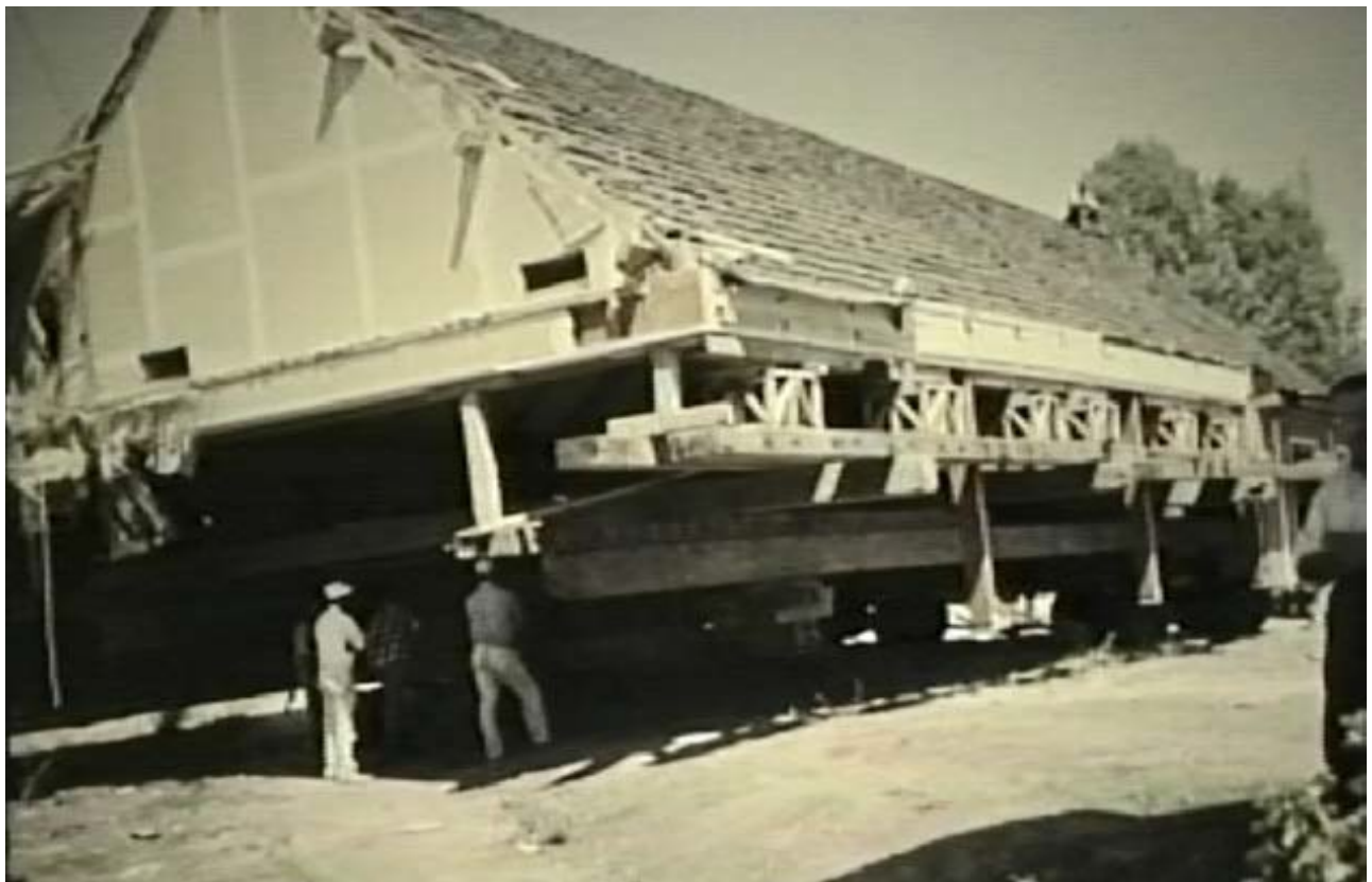
The house of prayer construction at Franklin Blvd.
